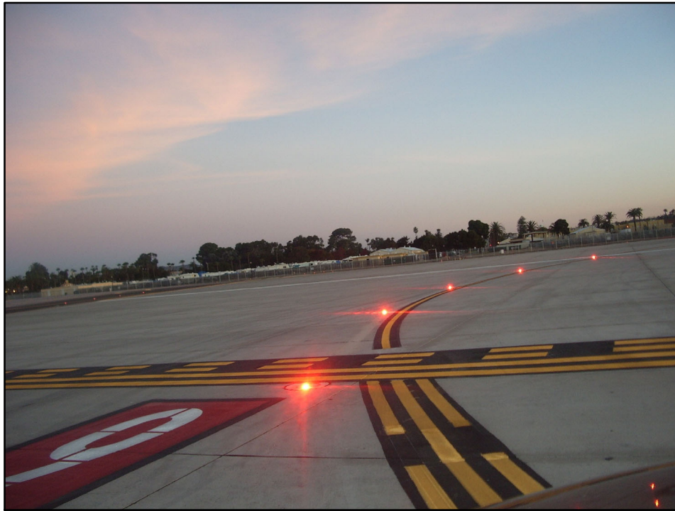
FIG 2-1-10 Runway Entrance Lights
